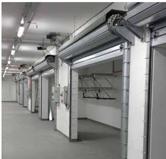
CURSTEEL, Data Center Orange - Val-de-Reuil
